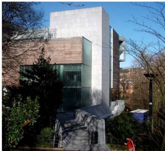
Figure 14 (Source: Conodate unpublished 2009). Glucksman Art Gallery, UCC with a floor area of 2,350m 2 . A 15°C single well, open loop system provides 190kW of heating and 130kW of cooling (Source: Kondwani et al. 2010).
