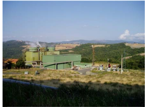
Figure 3. Larderello standard unit of 20MW dry steam electricity generating power plant – Italy (Source: SLR unpublished 2010).
