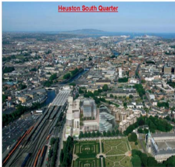
Figure 8. The Heuston South Quarter Development of 140,000 square metres of office space and 650 apartments was developed with district heating fuelled by its own 12MW energy centre supplied by a combination of wood pellet and gas boilers. If a geothermal heat source became available on economically attractive terms, this could provide the base load (Source: Architects Anthony Reddy Associates 2010; Building Services Arup Consulting Engineers 2010).
