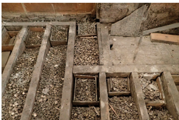
Boxes of shells placed between floorboard joists, used as soundproofing material
