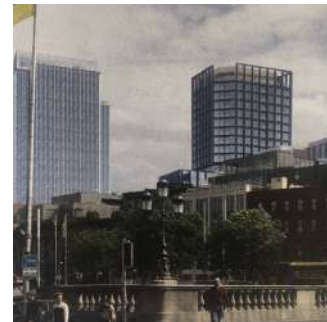
O'Connell Bridge, Dublin 1
