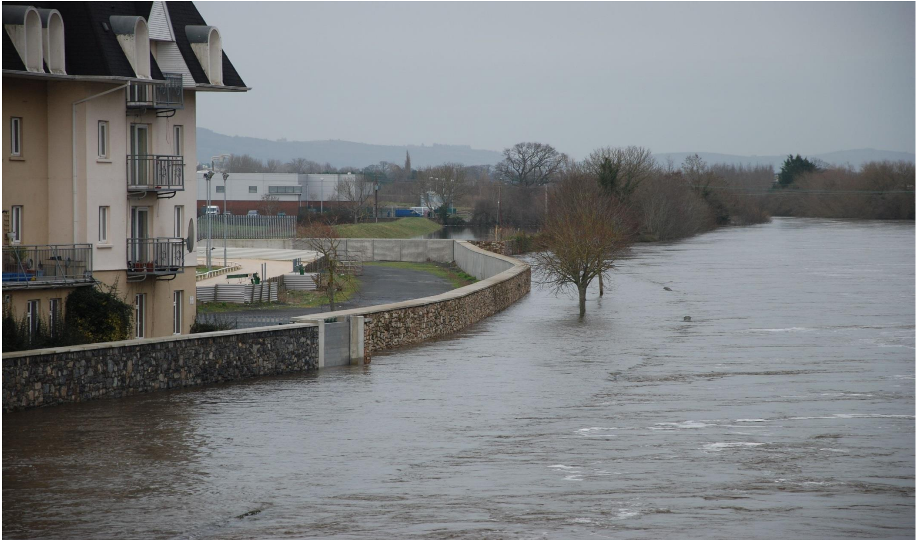
CLONMEL Flood event February 2014 (showing the flood well outside the normal bank)
