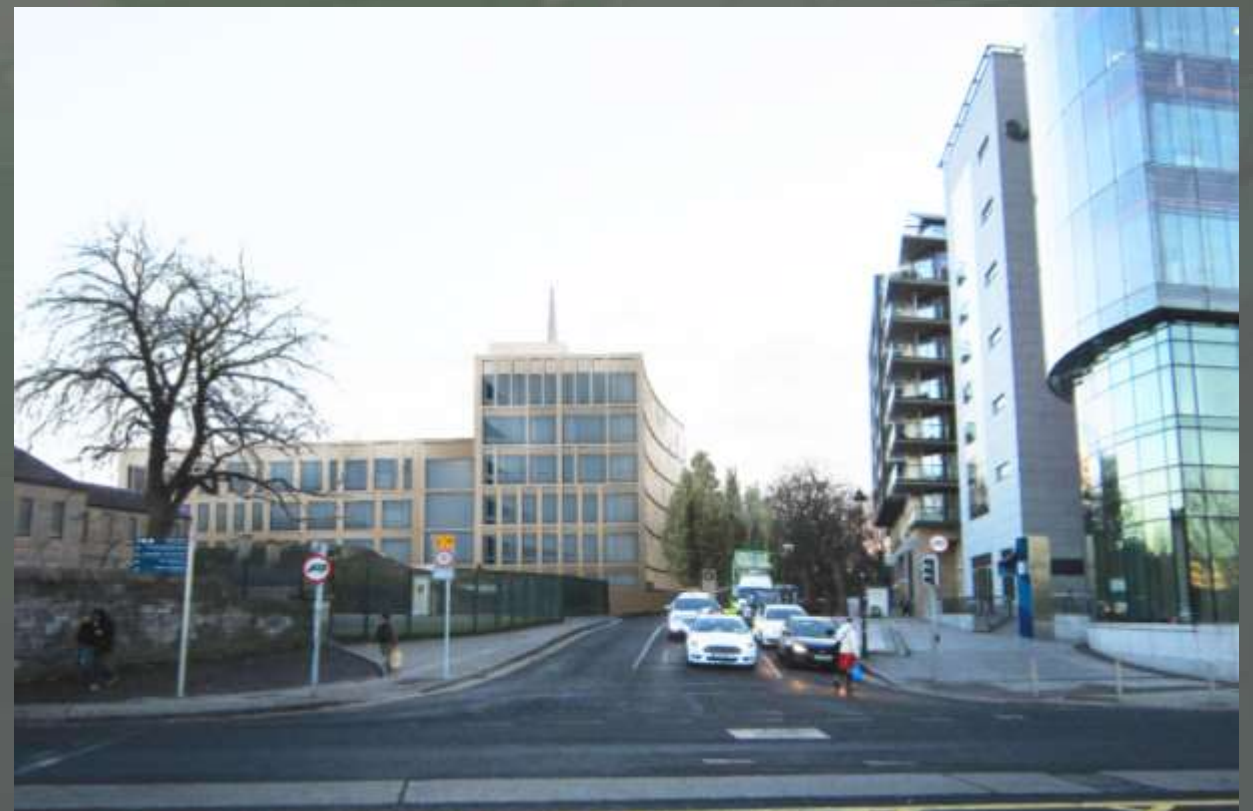
Garda Security and Crime Operations Centre, Military Road
